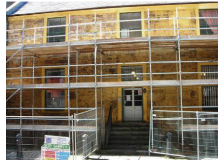
Phase II of building repairs are underway for August completion
